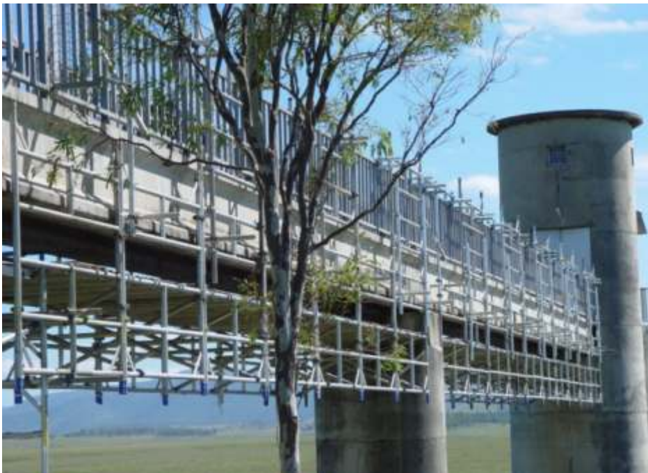
A Suspended Catch platform installed at Wivenhoe Dam.
