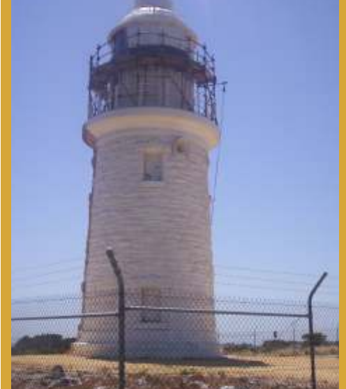
The Woodman Point lighthouse surrounded by scaffolding.
