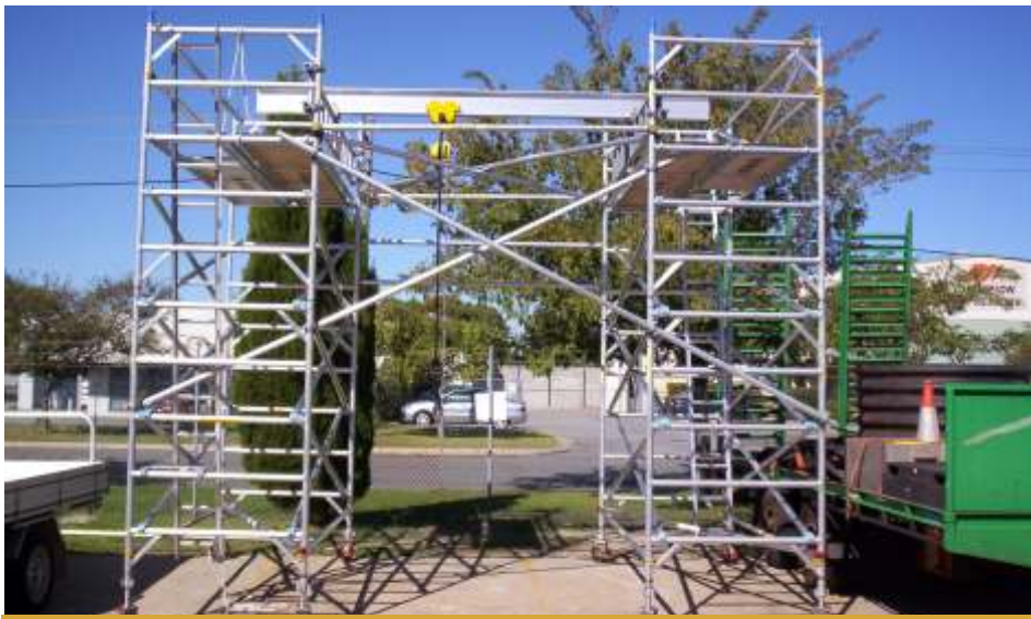
Mobile scaffolds assembled offsite
