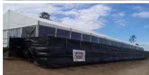
Scaffold and stage at V8 Super-cars Raceway
