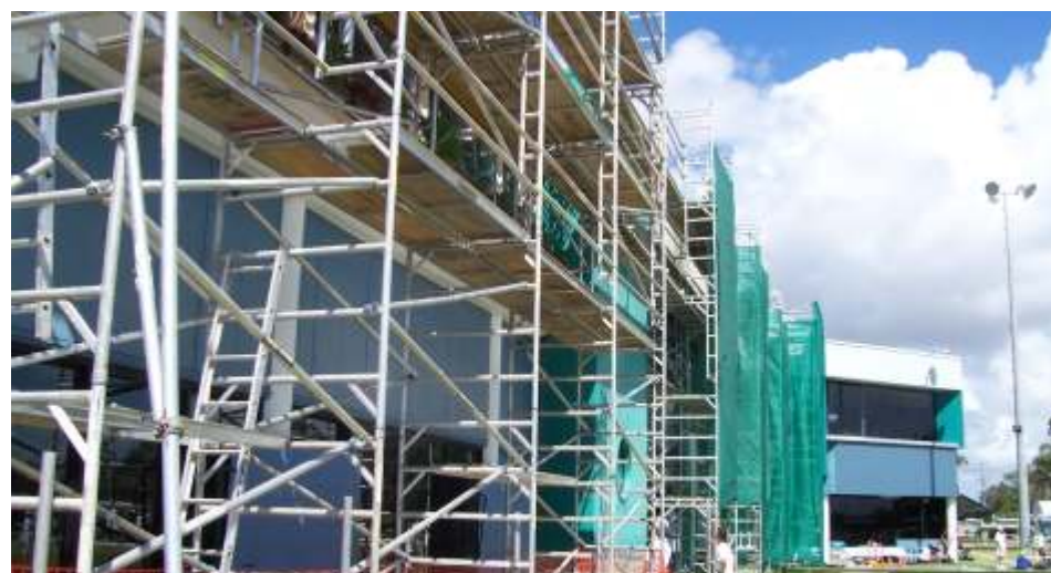
Scaffolding at Tweed Heads Bowling Club
